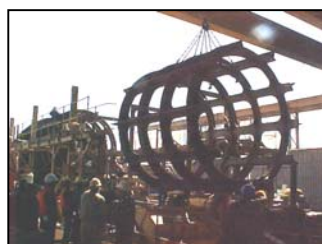
Old trommels being removed on site.
