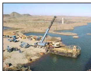
Crane loading barge with first part.
